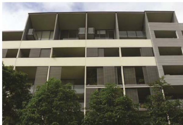
Photo K17-17 Deep balconies and adjustable screens shade windows from undesirable heat gain
